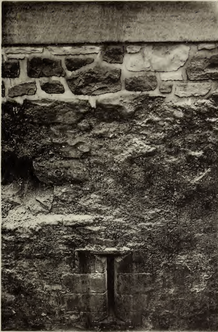
(FIG. 6) EXTERNAL FACE OF DAVID'S TOWER WHERE FIRST EXPOSED
